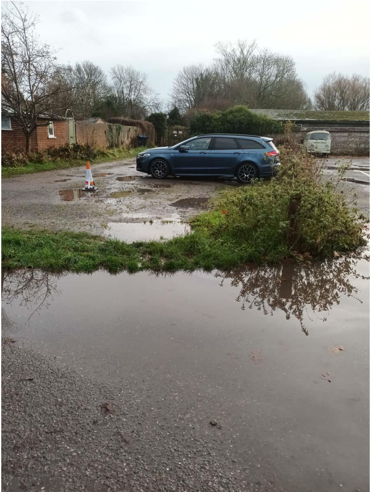
Flooding at the Entrance to the Car Park
