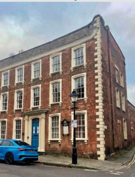
Chandos House, Bridgwater
